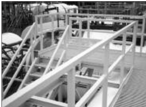
Handrail is used on walkways and platforms for safe maintenance free worker access.
