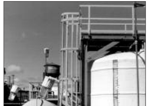
Fiberglass ladder cage assembly provides worker safe access to an outdoor platform.
