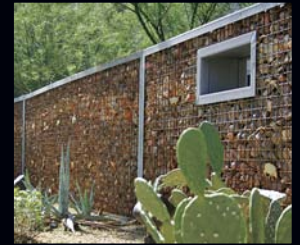
Rock Wall Fencing
